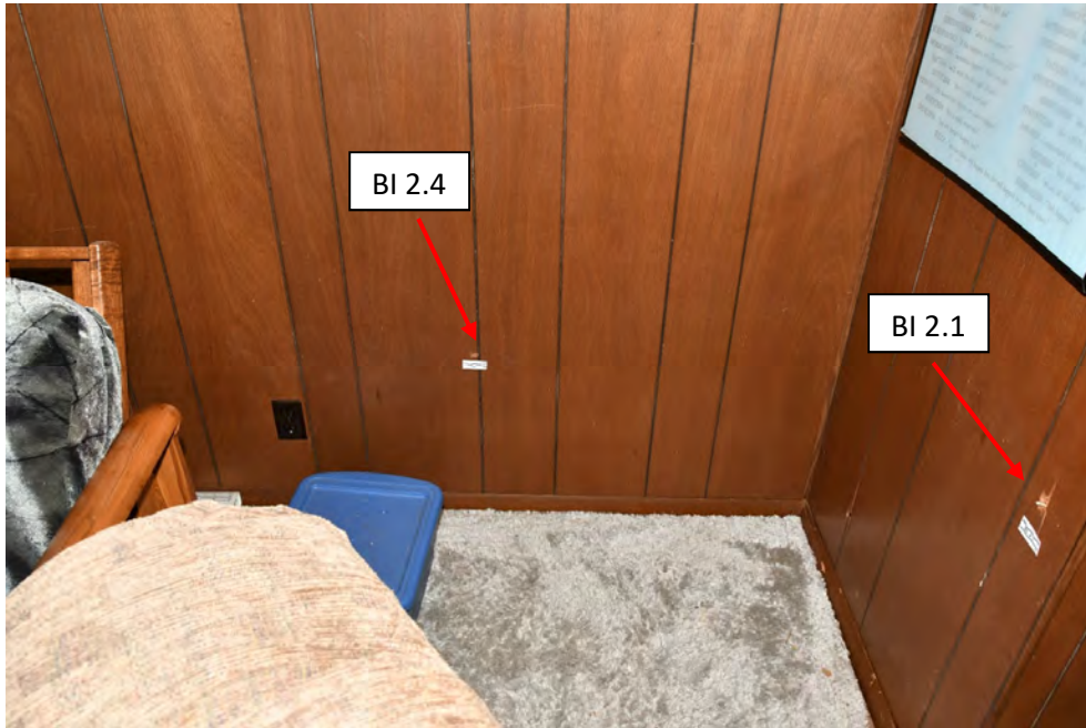
Figure #28 – Location of BI 2.4, West wall of living area
