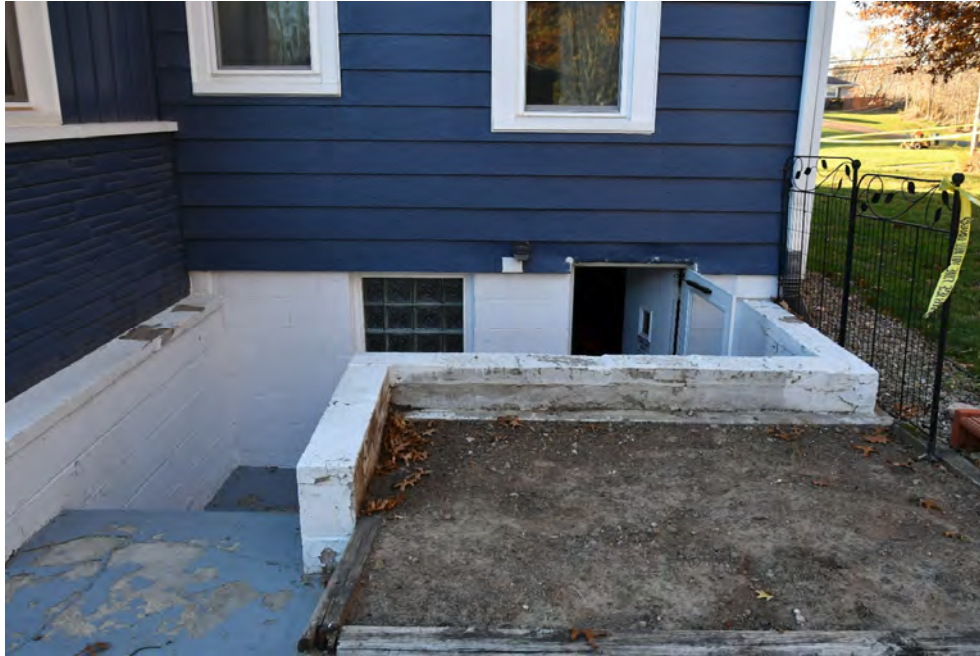
Figure #2 – Overall basement entrance from backyard
