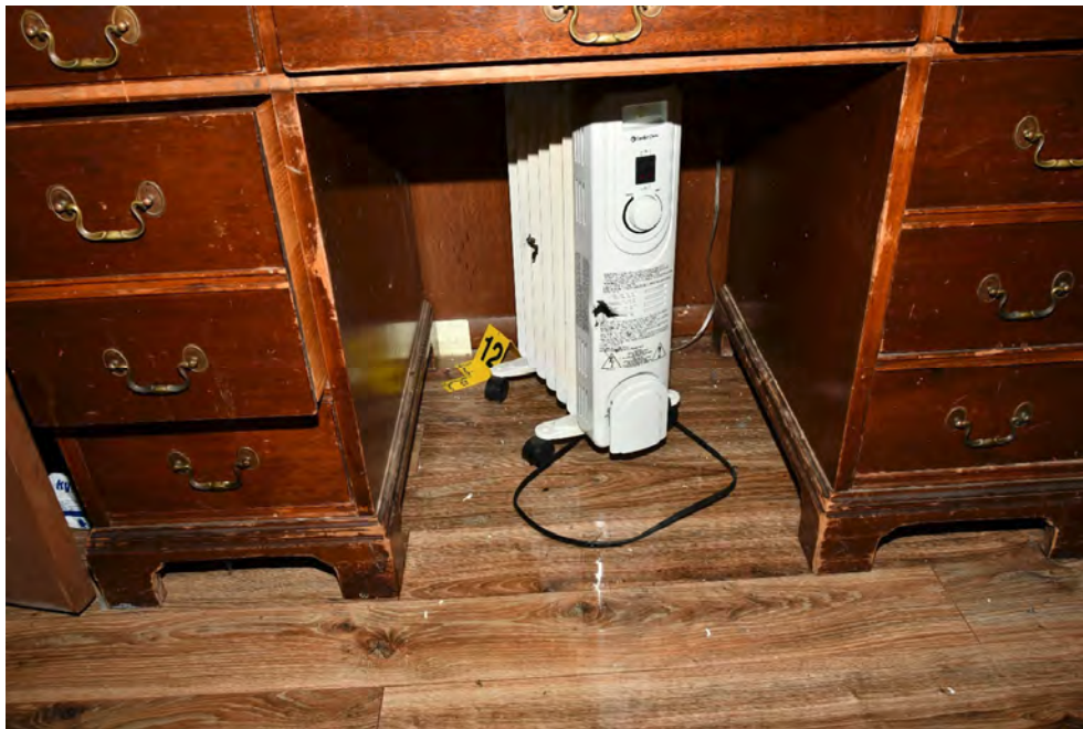
Figure #16 – Overall location of Item #12
