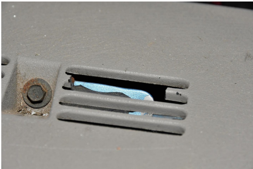
Figure #47 – Suspected ballistic impact to vent area next to BI 8.0
