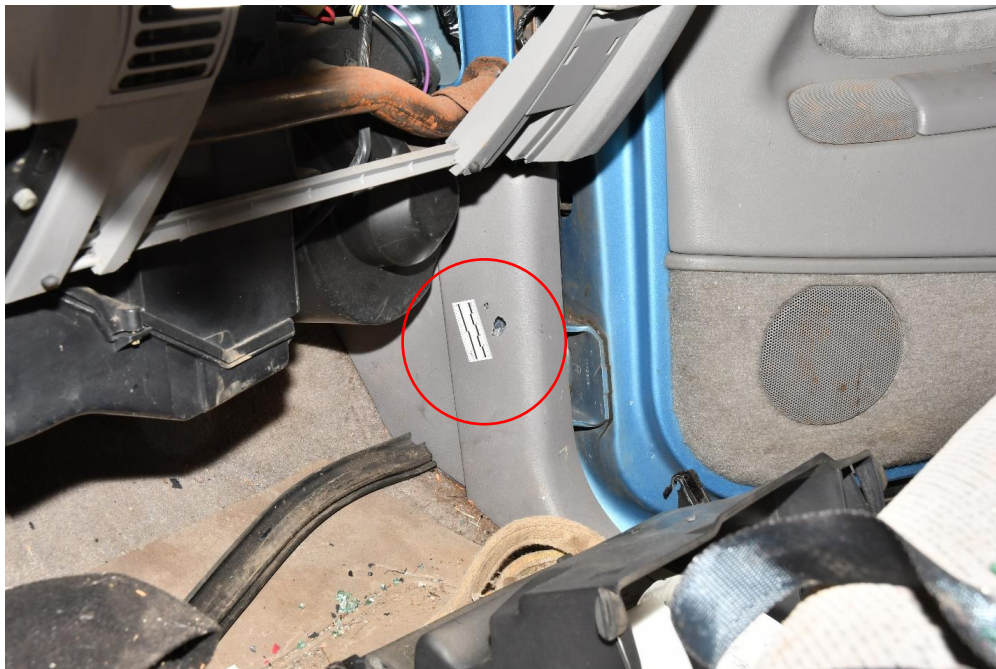
Figure #16 – Suspected ballistic impact, passenger floor column panel
