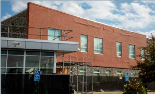
The brick and stone façade of Zane State's Advanced Sciences and Technology Center is splitting and crumbling on three sides due to problematic design and construction, AG Yost's lawsuit maintains.
