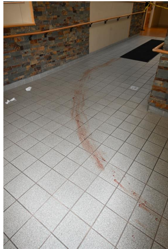
Ramp in Emergency Room
