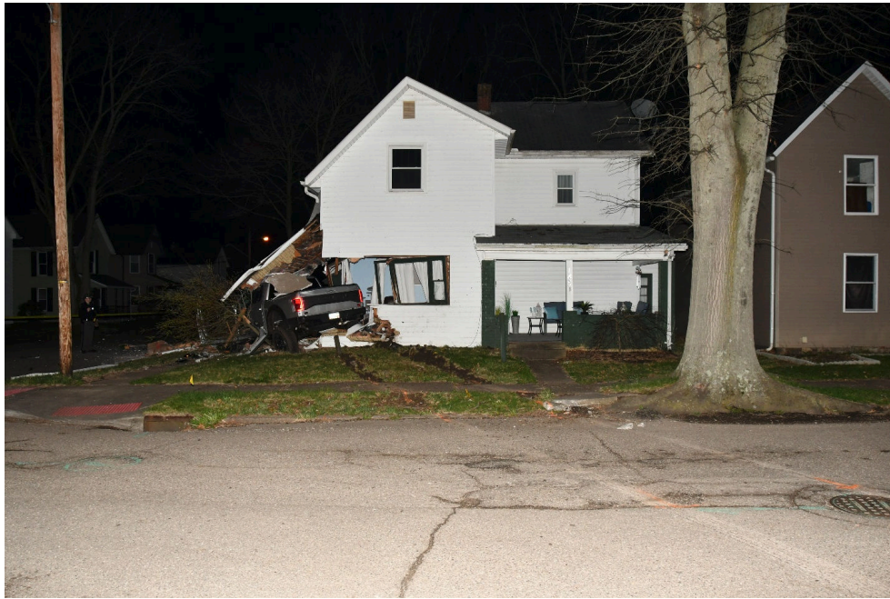
Figure #2 - Front Exterior 145 8 th Street NE
