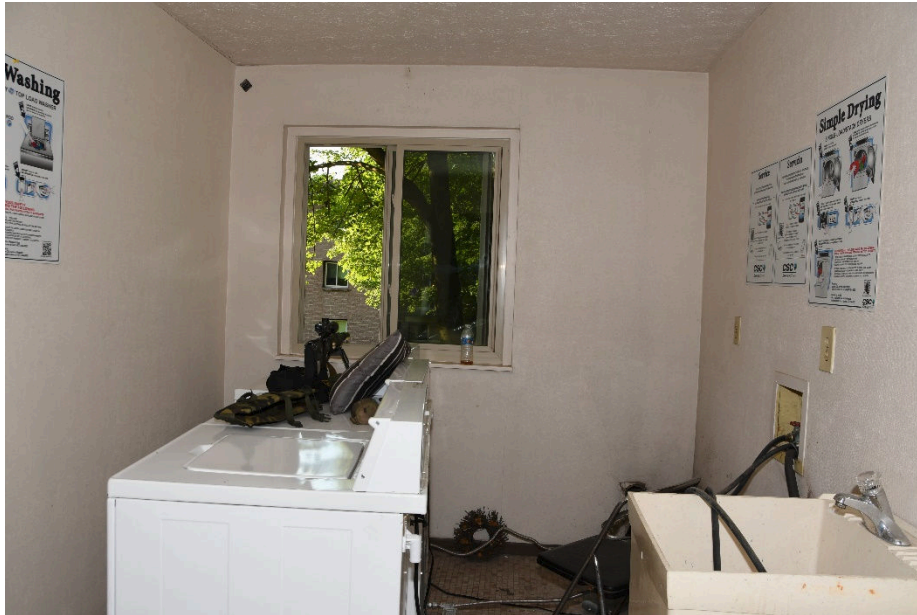
Figure 1, Laundry Room Overall
