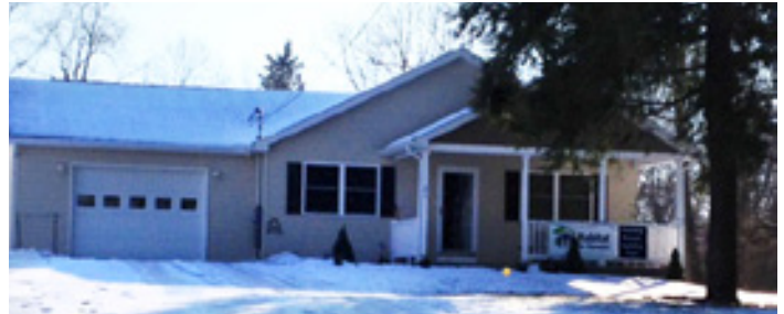
A new house built by Knox County Habitat for Humanity in Mt. Vernon, Ohio.
