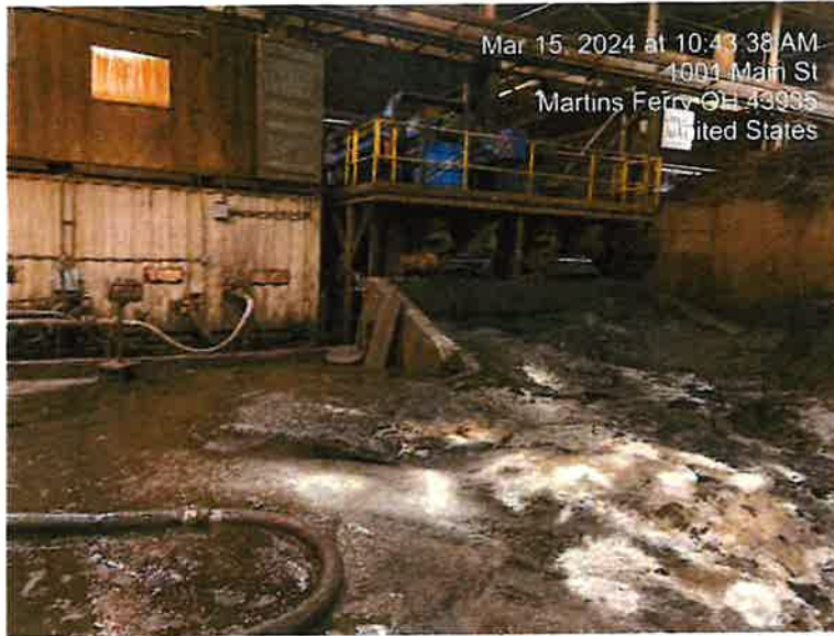
Filter press solids storage area
