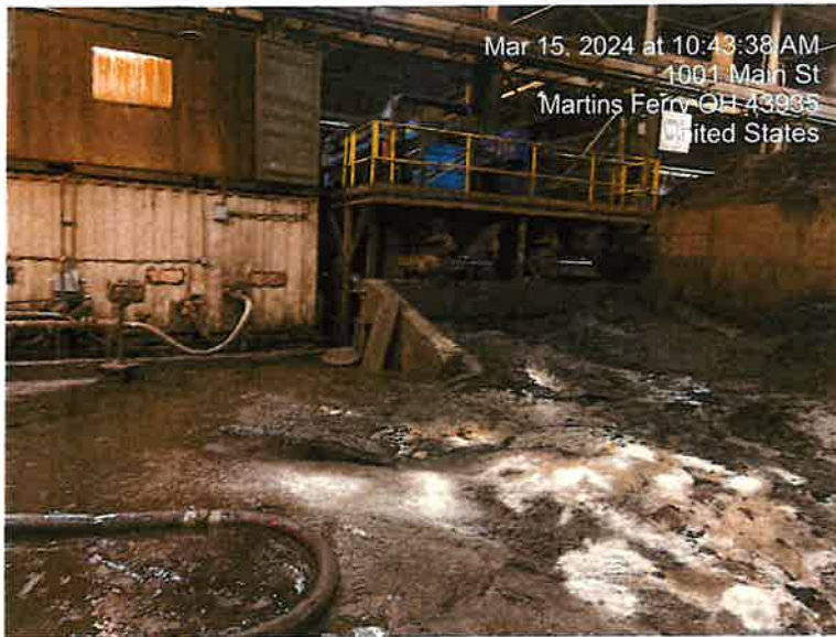
Filter press solids storage area
